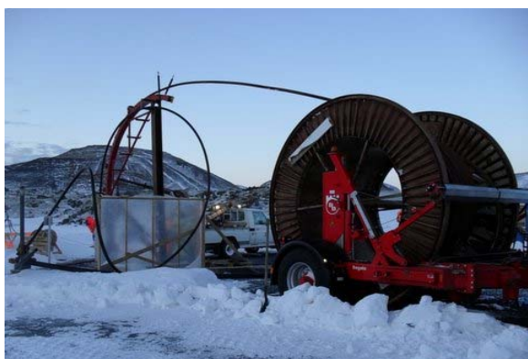
Figure 4 – Installation of downhole pumps in monitoring wells in November 2009. Photo: Þorsteinn G. Kristmundsson
