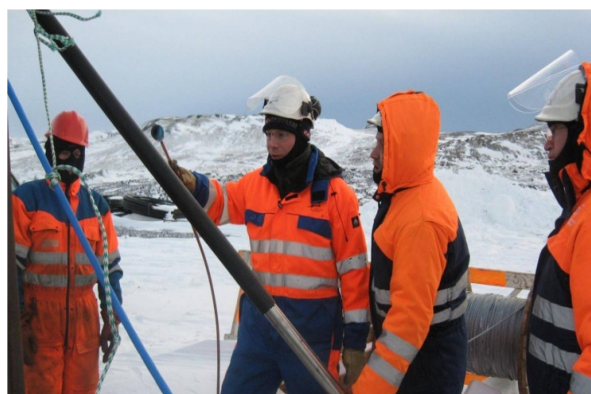
Figure 4 – Installation of downhole pumps in monitoring wells in November 2009. Photo: Þorsteinn G. Kristmundsson
