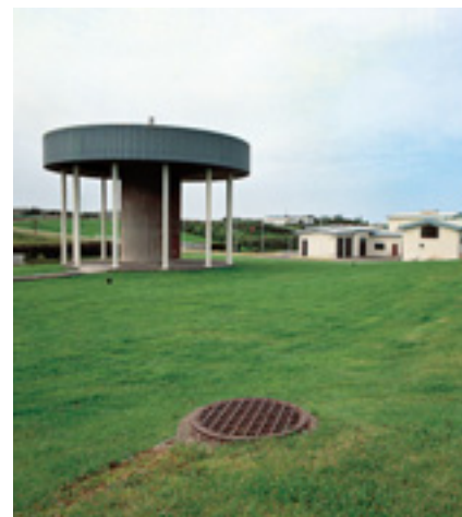
Pumpingstation at Reykir Mosfellsbær.
