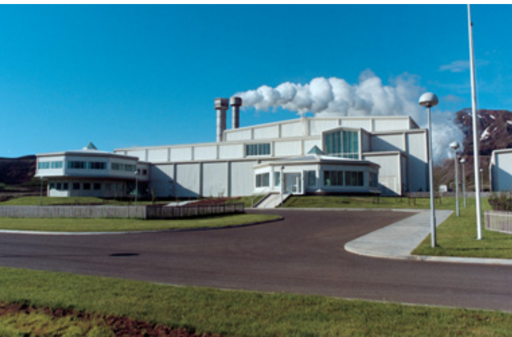
The power plant at Nesjavellir.
